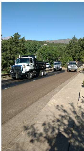
Repaving north Golden Hills Rd.
