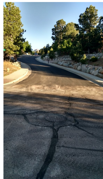
Repaving Flatrock Place
